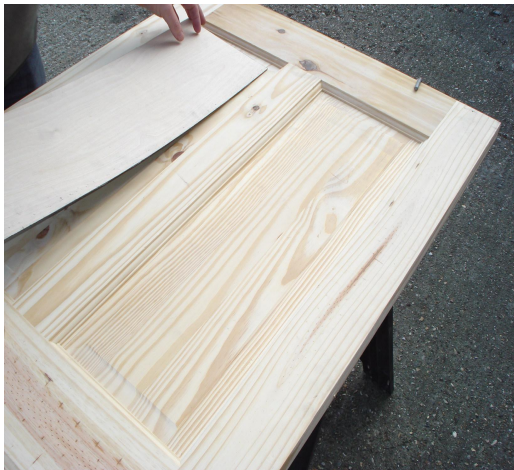
Pyroplaque being applied to thin door panels
