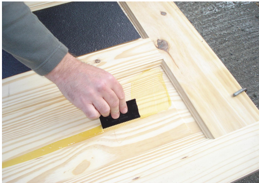
Pyroplaque being applied to thin door panels
